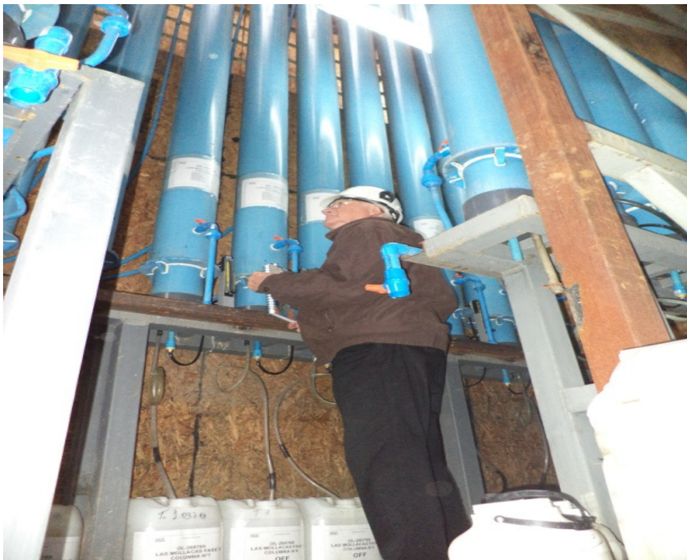
Figure 6: Mollacas 6 metre columns at the SGS laboratory in Santiago, Chile
